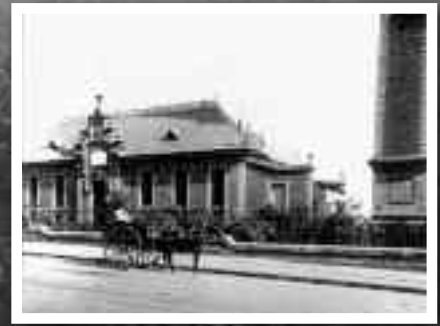
Above: Crown Street Pump Station 1876
