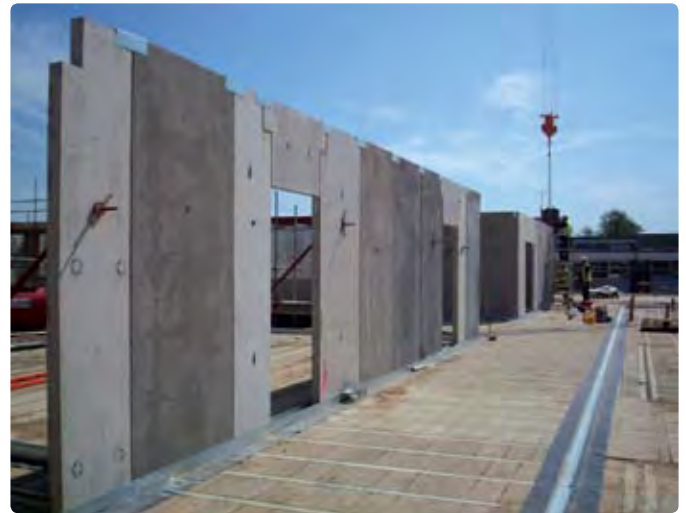
Figure 2 left: Fastbuild panel being lowered into position.
