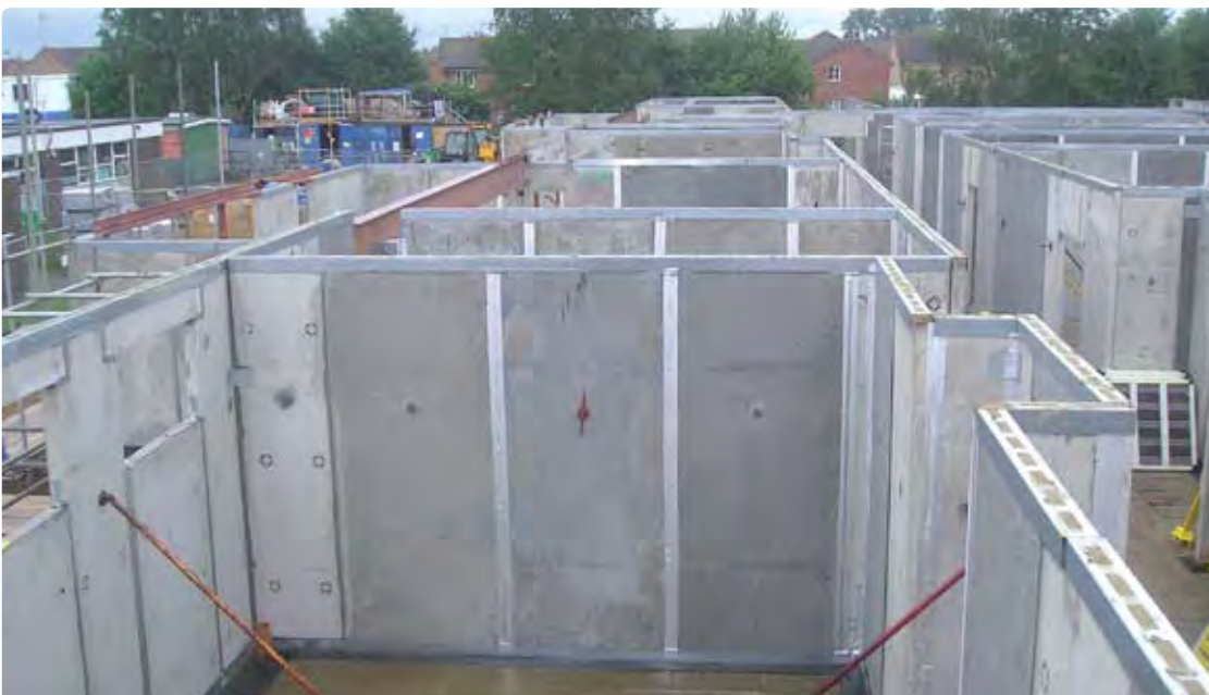
Figure 4: Panels propped in position to form classrooms and corridors.
