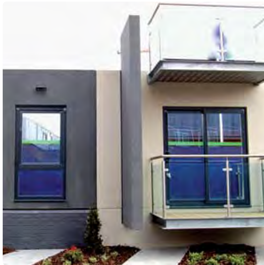
Figure 2 right: Built as one complete unit, PCE's system incorporates precast concrete façade and wall panels, fenestration, insulation and exterior features 'all in one'.
