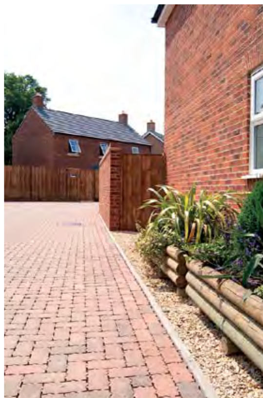
Figure 1 right: Domestic parking areas installed with Brett Omega-Flow paving reduces the burden on highway drains and sewer systems.
