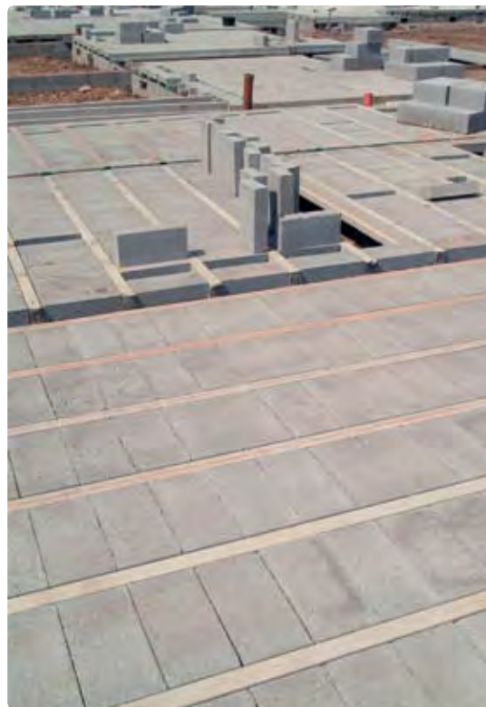
Figure 4: CEMEX beam-and-block flooring at ground-floor level on a residential site.
