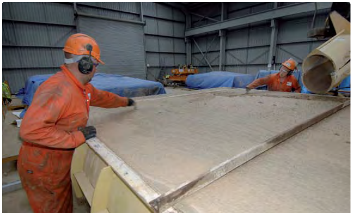
Figure 1: Pouring a revetment element.
