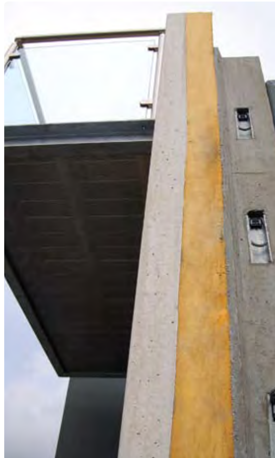
Figure 1: A section through the sample panel showing the precast concrete and insulation ‘sandwich’ along with the integral balcony.
