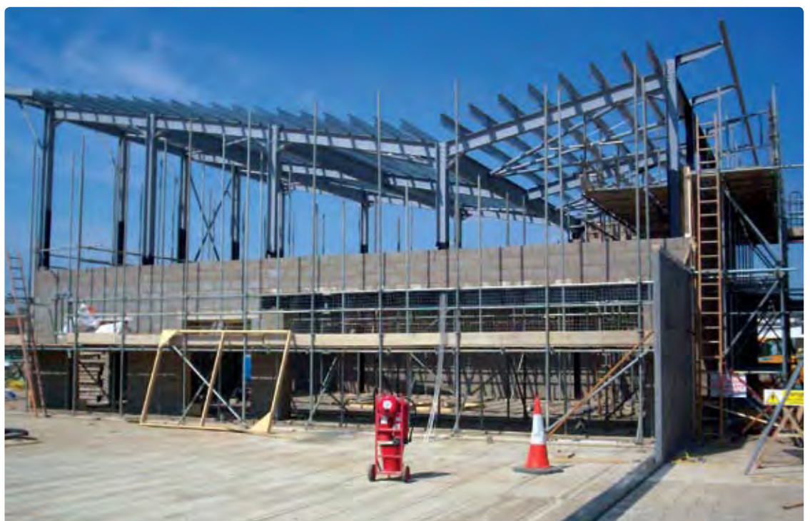
Figure 1: Fastbuild panels integrated with steel frame.
