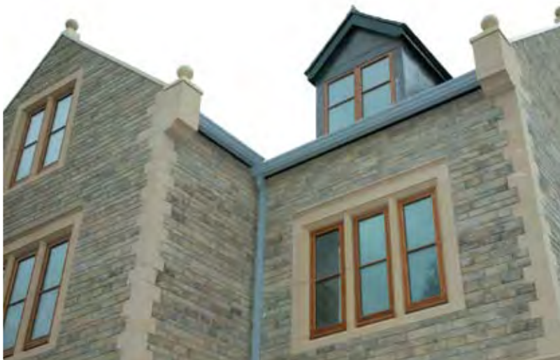
Figures 4 and 5: The project aim was to retain the intended visual appearance and harmony of the original house. Bradstone's walling range, cast directly from hand dressed natural stone masters, was used for this effect.
