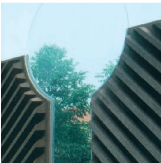
A profiled concrete absorptive barrier with tree-shaped acrylic windows. The granular concrete is highly profiled to maximise the noise absorption.
