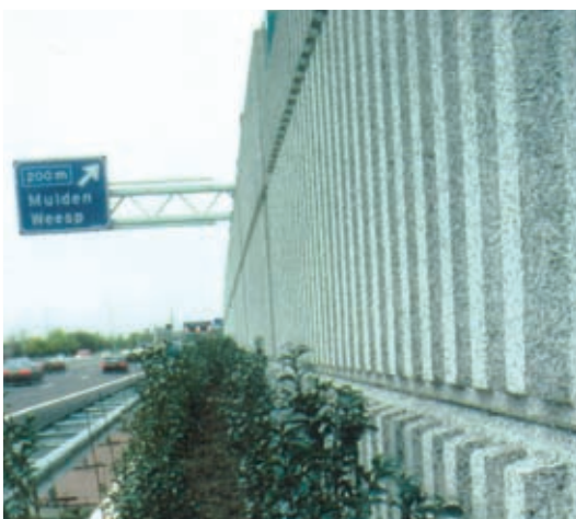
Profiled wood fibre concrete, an example of an absorptive barrier.
