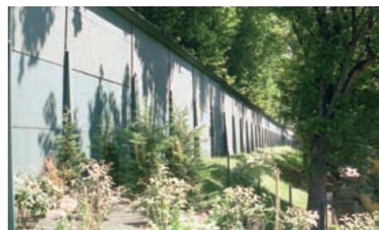
Painted green on the traffic side to match the plane trees, this precast barrier near Paris incorporates sound absorbent concrete and an anti-diffraction coping.
