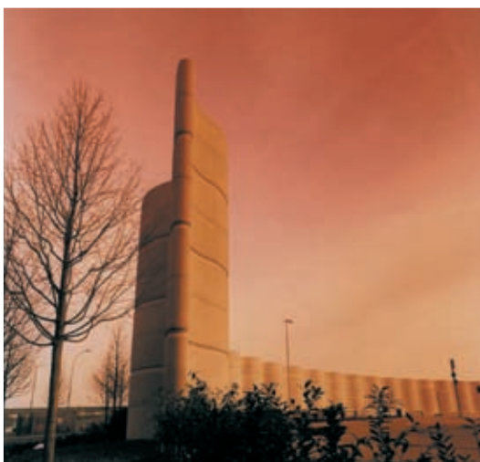
The wave wall at Gatwick contains noise and blast from manoeuvring aircraft.
