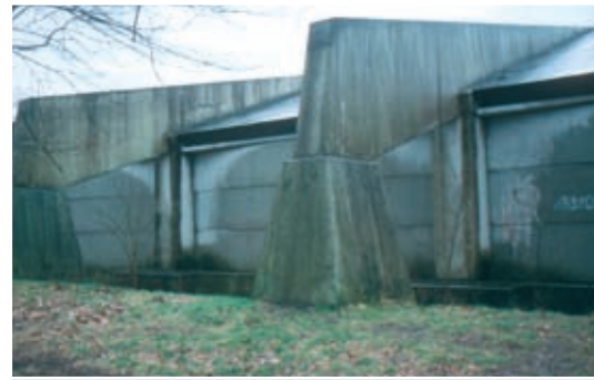
This large concrete barrier that cantilevers over the hard shoulder of the A28 motorway at Zeist in the Netherlands protects the adjacent housing estate from the traffic noise.
