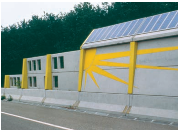
The sunray motif used at the end of this barrier in Utrecht, The Netherlands, signals that the barrier supports solar panels.
