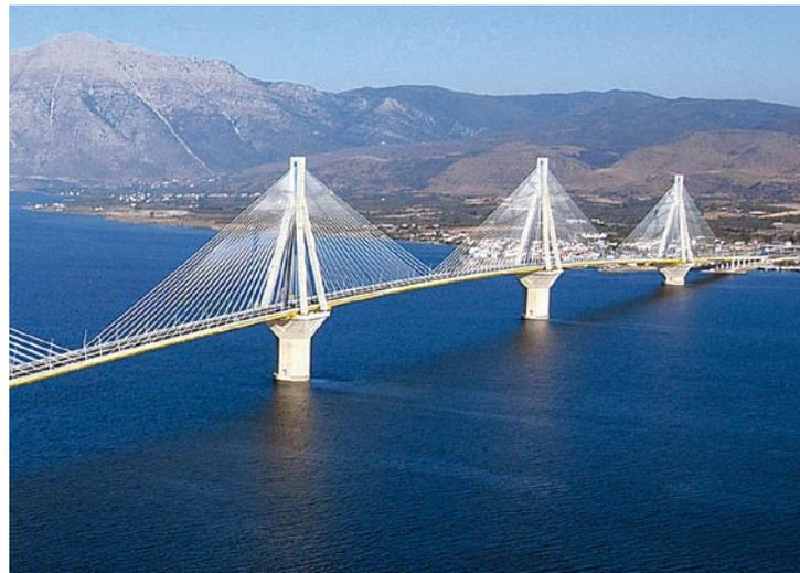
The 'Rion-Antirion' suspension bridge in Greece is a structure that calls for a long service life. The bridge is 3km long and the centre span is 560m long. Courtesy of FIB.
