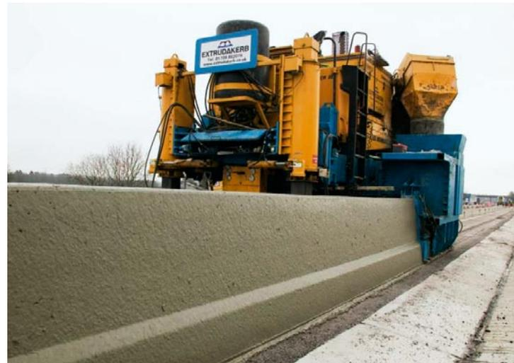
Concrete safety barrier now being used on all motorways. They are designed to achieve an essentially maintenance-free serviceable life of not less than 50 years. Courtesy of Britpave
