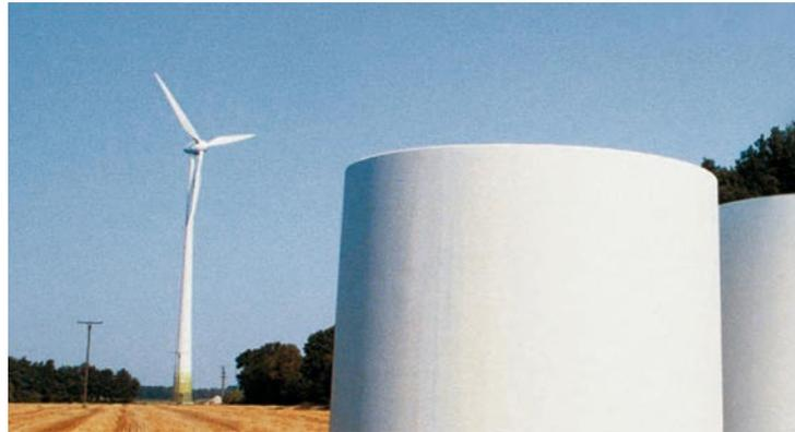
Precast concrete is often used for wind turbines - its high level of weather resistance and inherent stiffness help provide a stable and resilient structure that generates electricity, which is a renewable resource. Courtesy of the British Precast
