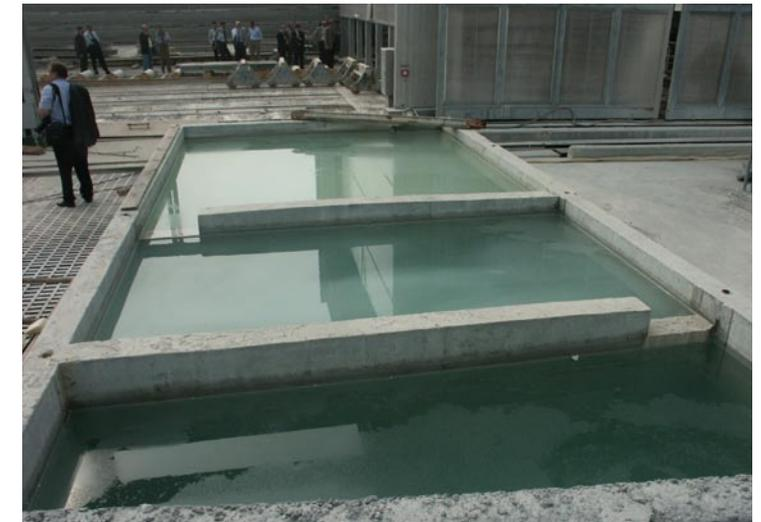
The solid material in process water in the concrete industry is allowed to settle out so the water can be recycled for concrete manufacture. Courtesy Betoni, Finland
