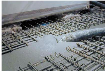
Self-compacting concrete is extremely fluid. It needs no vibration to compact and is easier to place, which is better for workers' health and safety and saves time.
