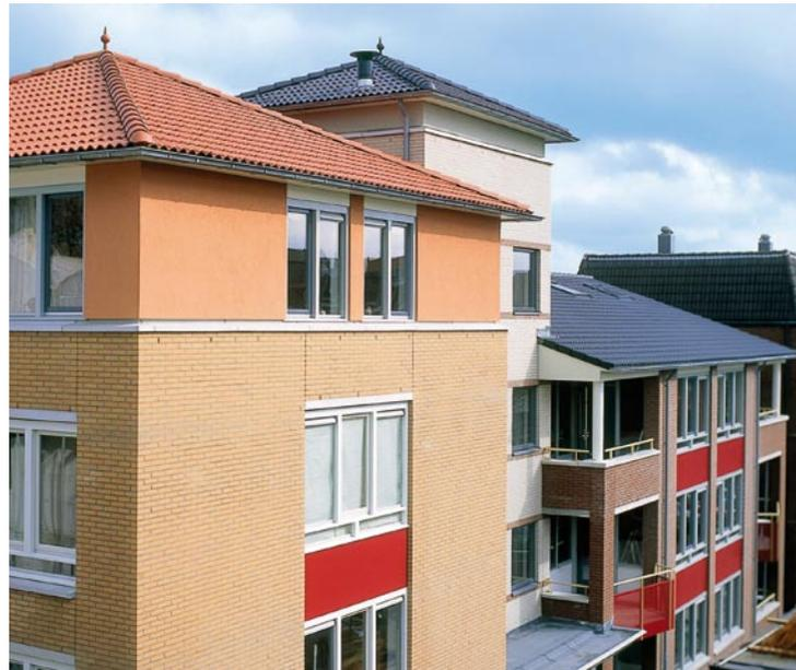
Dutch buildings made of precast concrete units. The concrete roof tiles used for the roof finish ensure a long service life for the building. Courtesy of BFBN.
