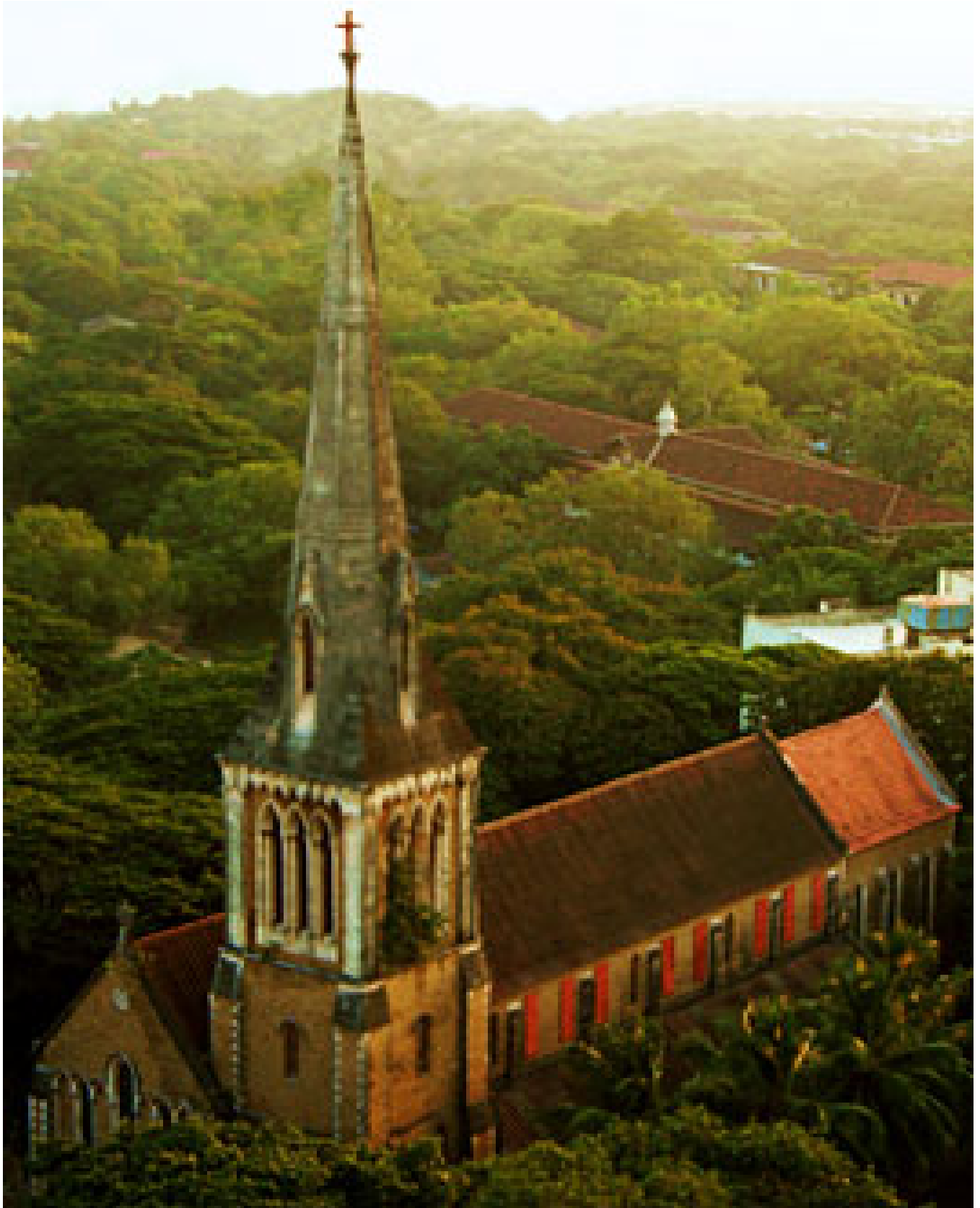
Aerial view of the Church of St John the Evangelist, better known as the Afghan Church
