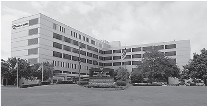
One of the two VA hospitals in Augusta
